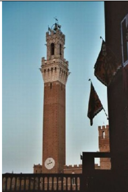
Top of the Torre del Mangia, the bell tower of the Palazzo Pubblico. The tower was completed in 1348 and is made of brick topped by a belfry of white travertine marble.
